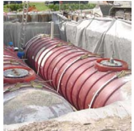
PETROLEUM TANK INSTALLATION
