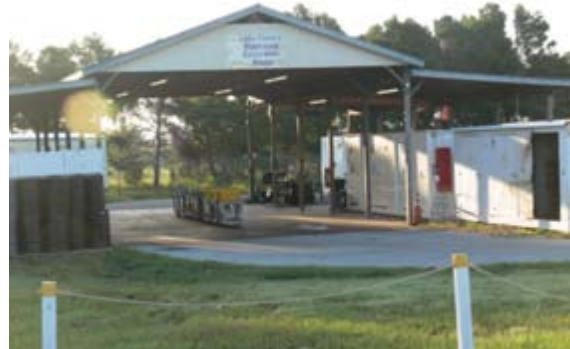
HOUSEHOLD HAZARDOUS WASTE FACILITY
